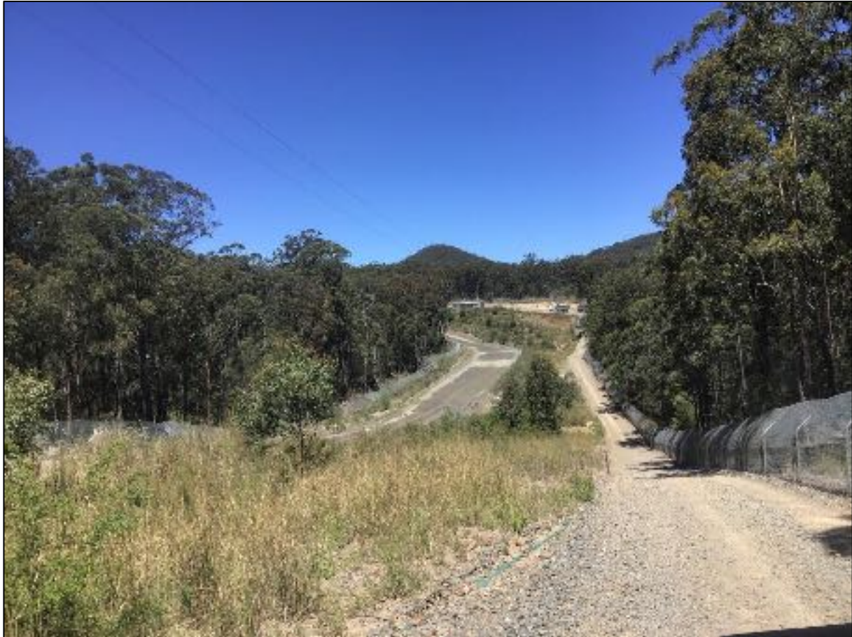
Plate 2: Sediment fencing along the light vehicle road
