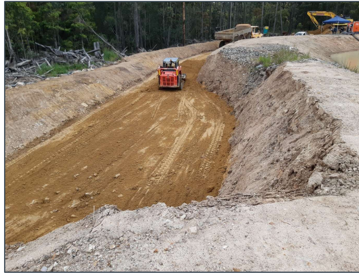
Figure 18: Dam wall remediation project
