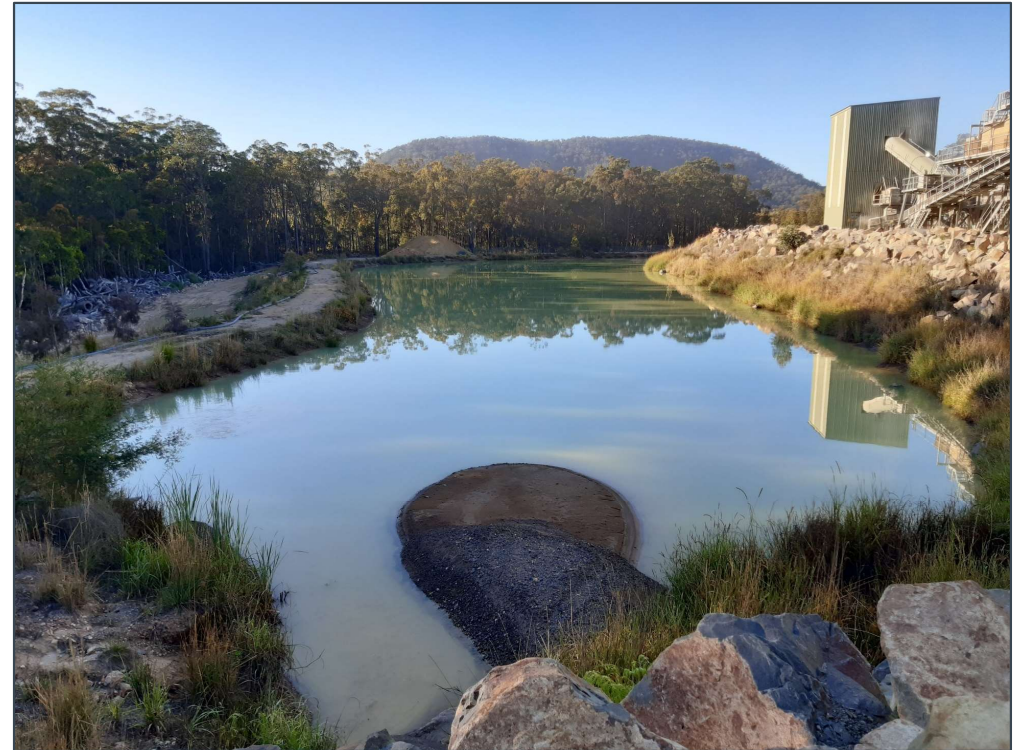
Figure 9: Dam 1 7:25am 27 October 2021
