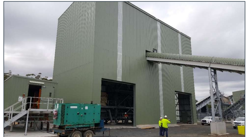
Figure 4: KEQ Secondary (Cone) Crusher Enclosure
