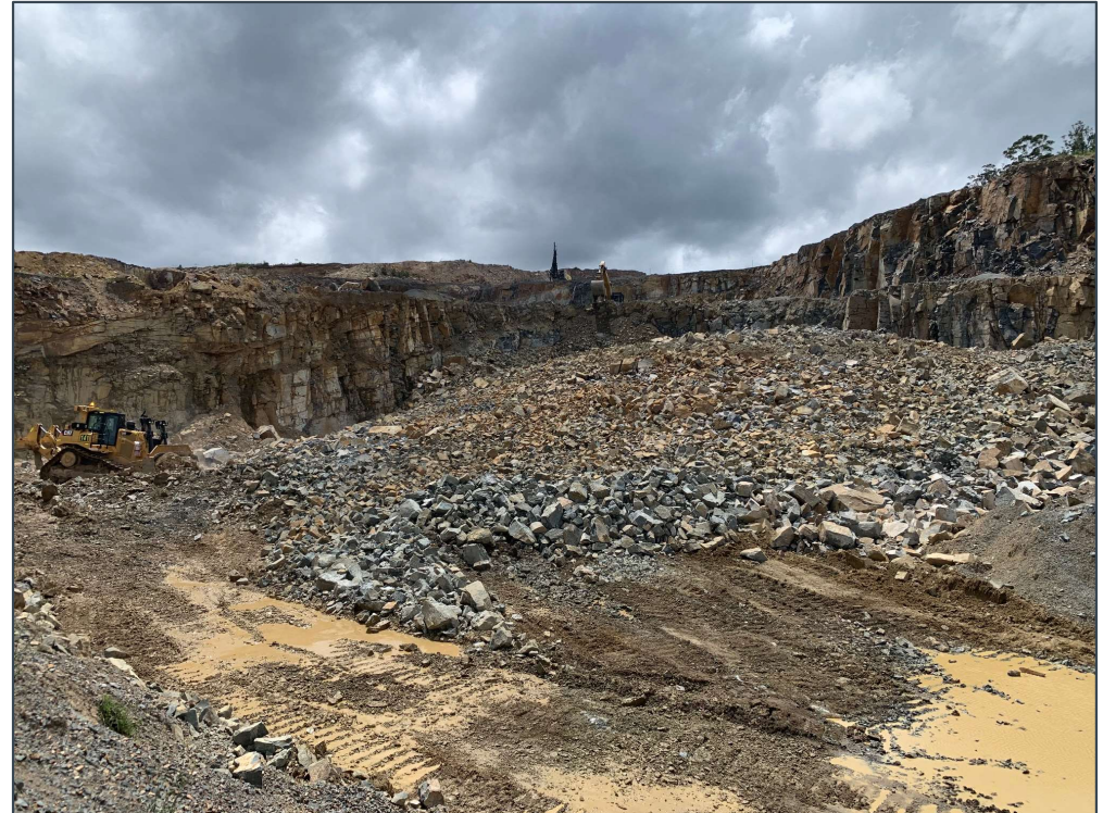
Figure 15: Post blast photo
