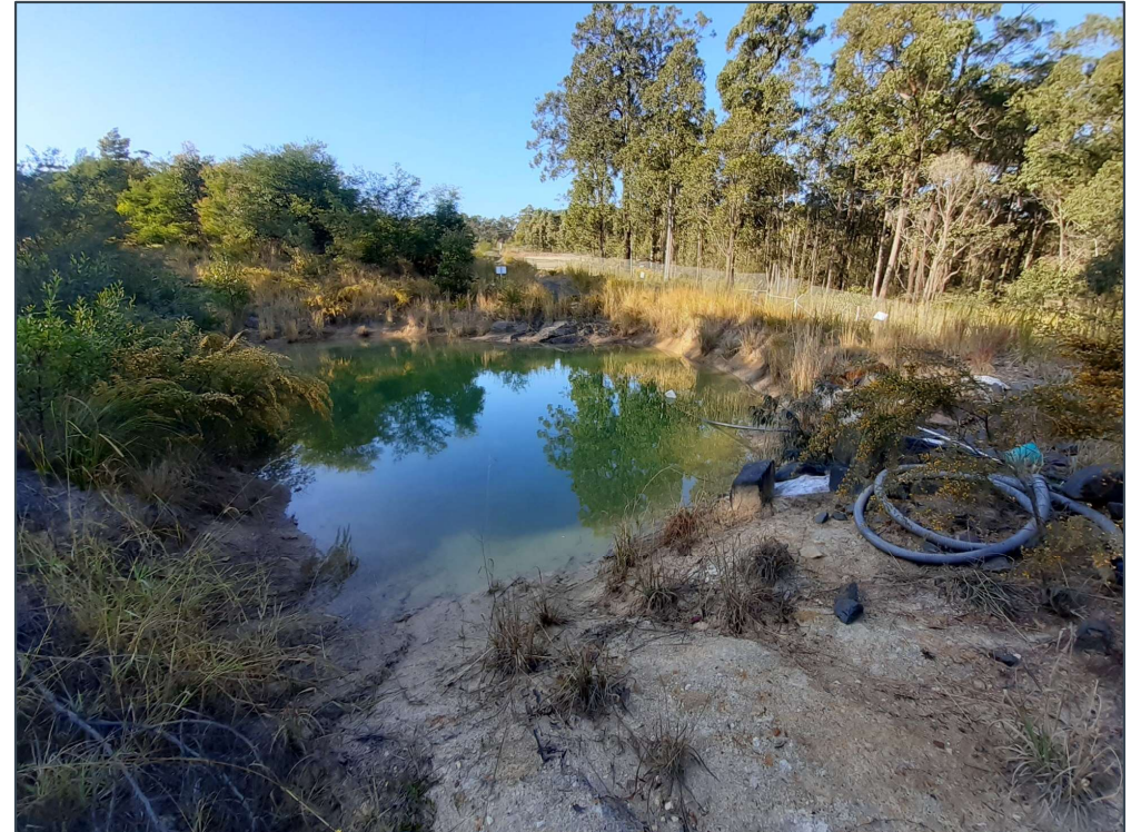
Figure 10: Dam 2 7:50am 2 September 2021
