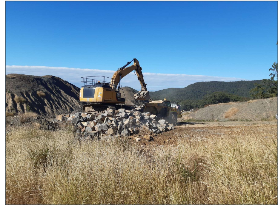
Figure 16: Excavator loading Class 2 into dumpy
