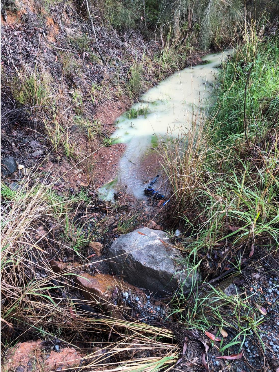
Photograph D.9 Sediment dam discharge point outlet
