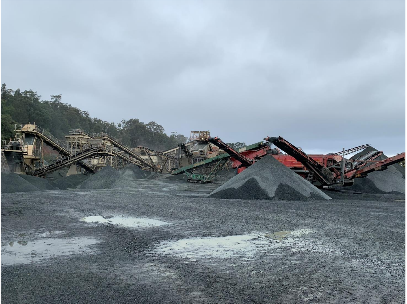
Photograph D.5 Crush and stockpile area
