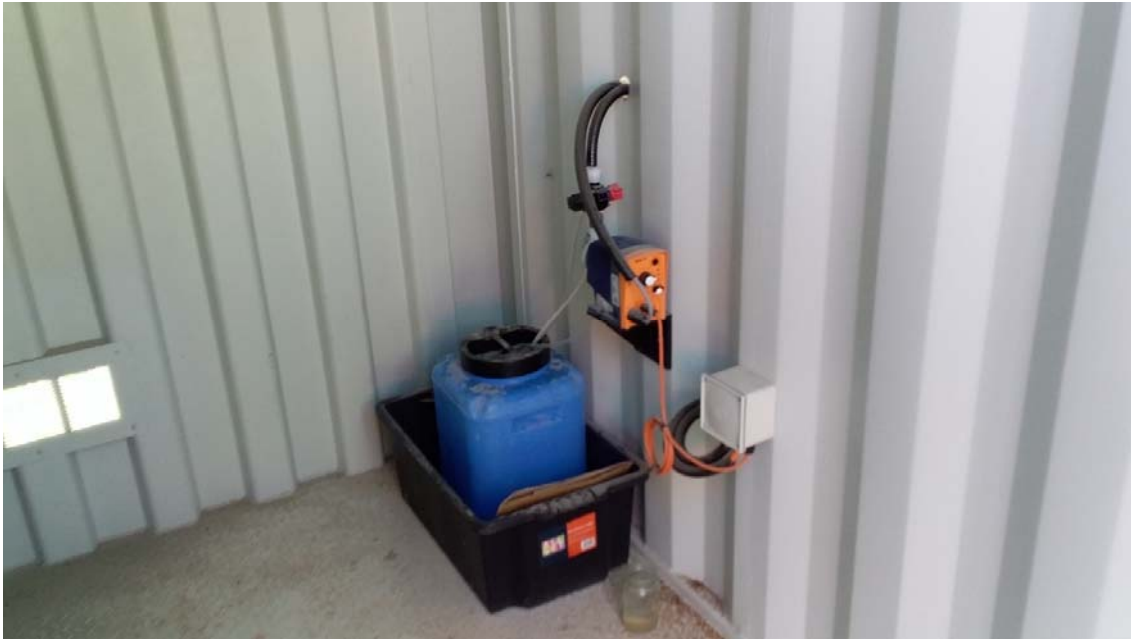
Plate 9 Dam 1 Flocculant Treatment System
