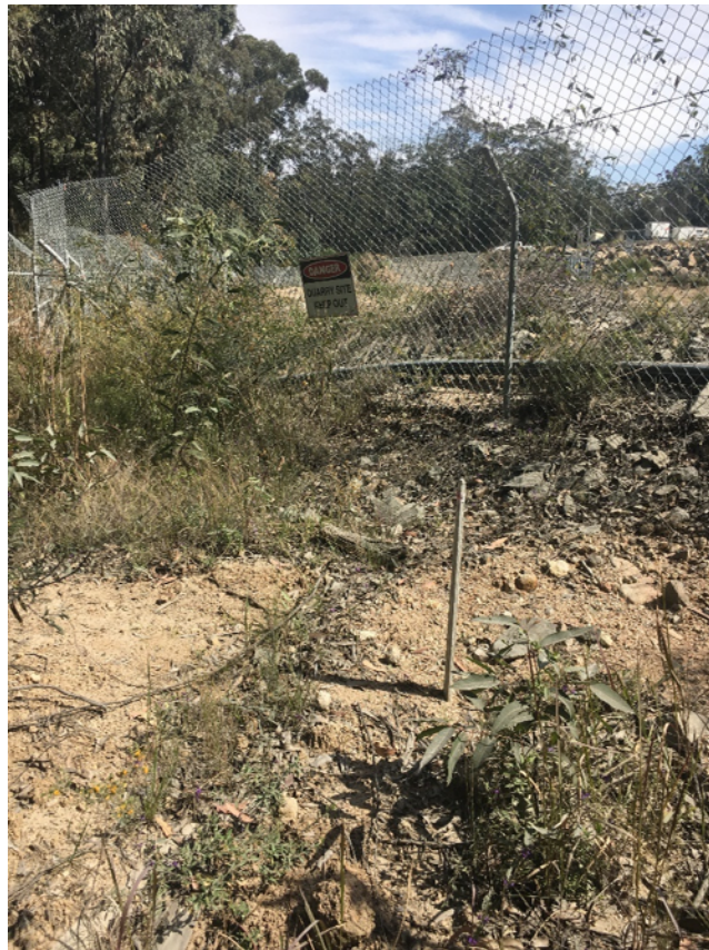
Plate 1 Example of survey pegs delineating site disturbance boundary
