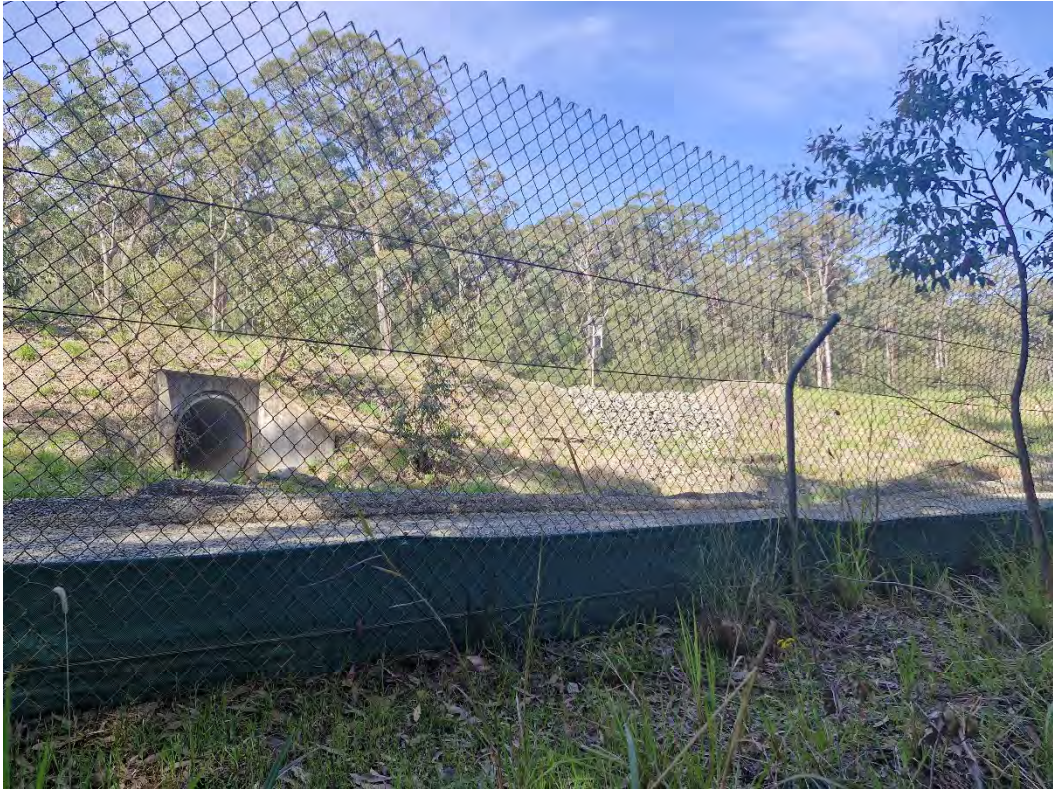
Photo 10: Sediment fencing repaired since previously damaged.
