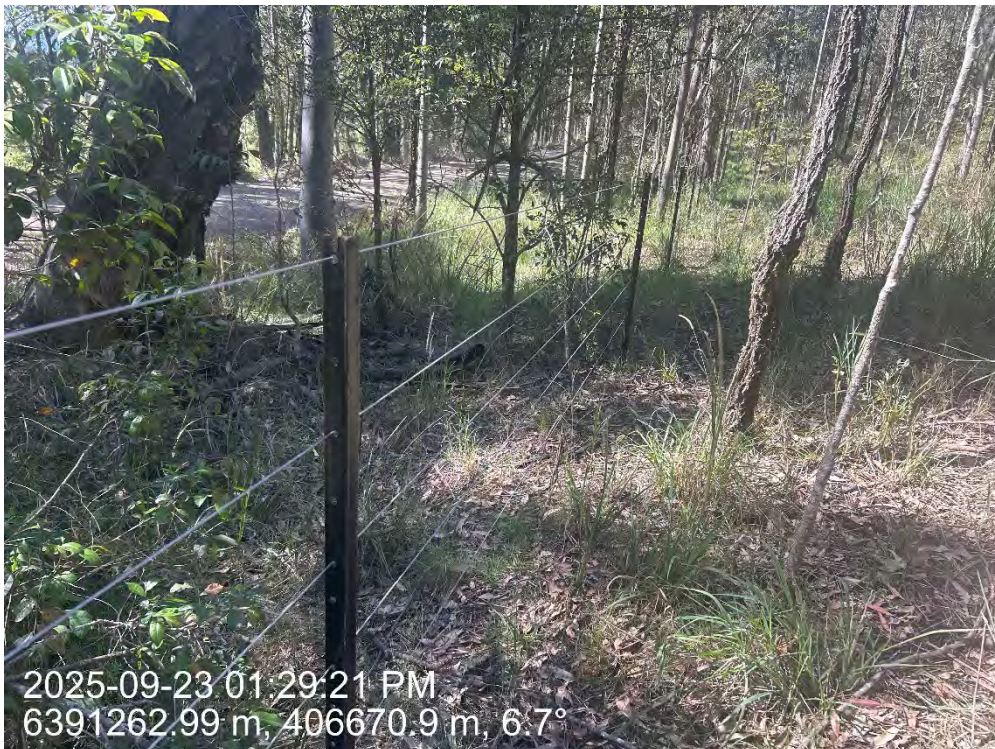
Photo 5: Fence repair works observed along far northern boundary in 2025
