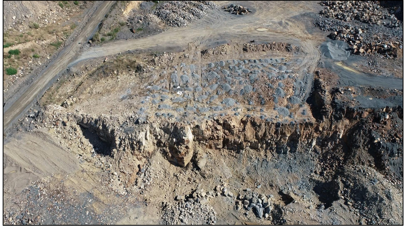
Figure 17: Post blast photo
