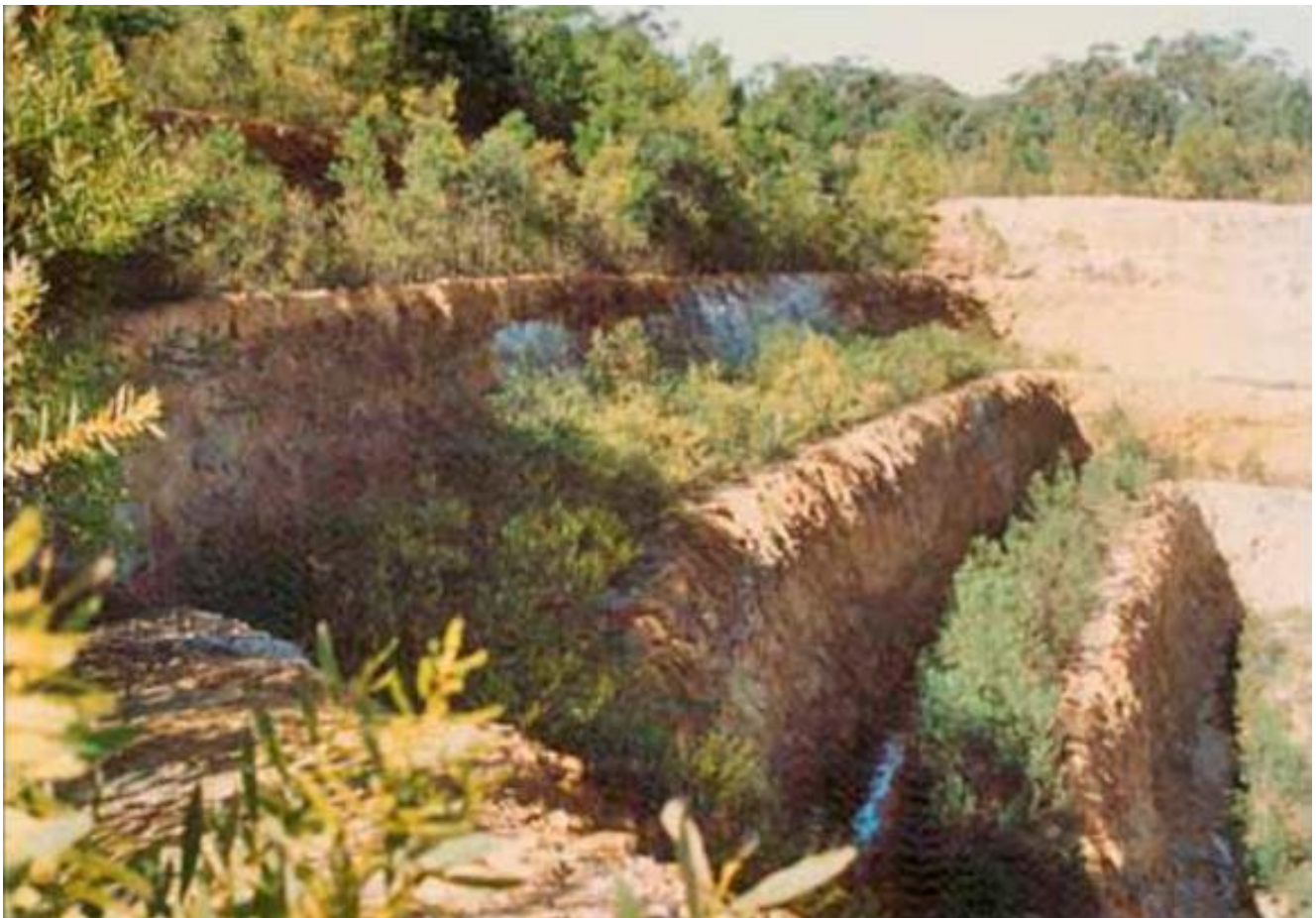
Figure 5 Example of Bench Rehabilitation.
