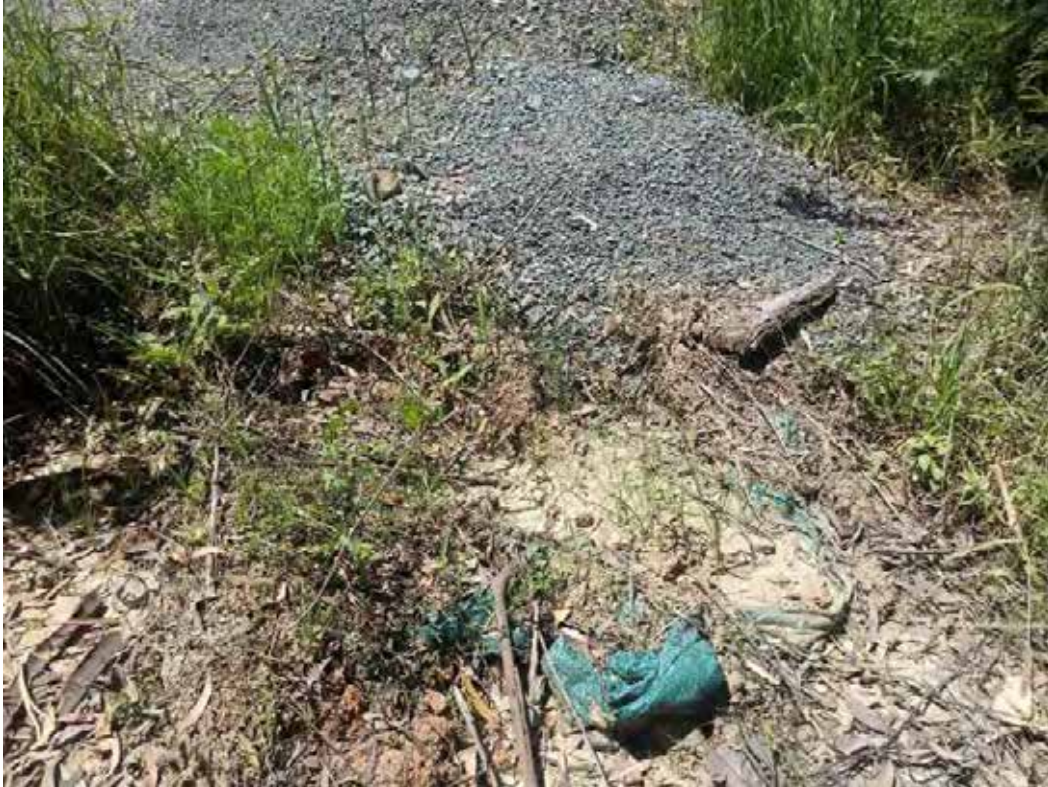
Photo 9: Sediment fencing down and overtopping within Lot 12.
