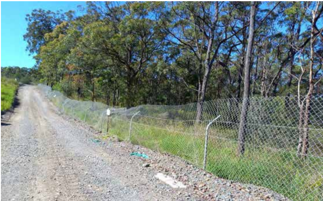
Photo 5: Fixed fence along western boundary of haul road
