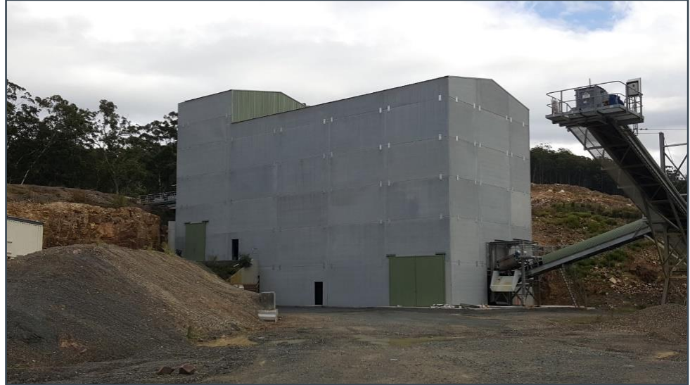
Primary Crusher Enclosure
