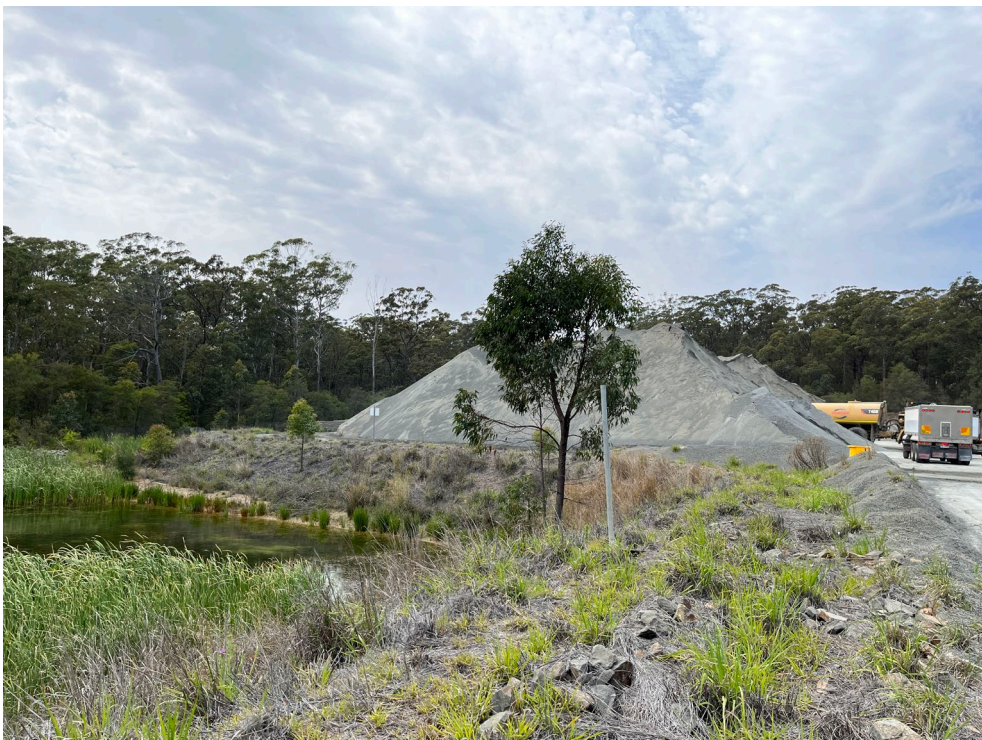
PHOTO 8 Product Stockpiles and Surface Water / Sediment Dam
