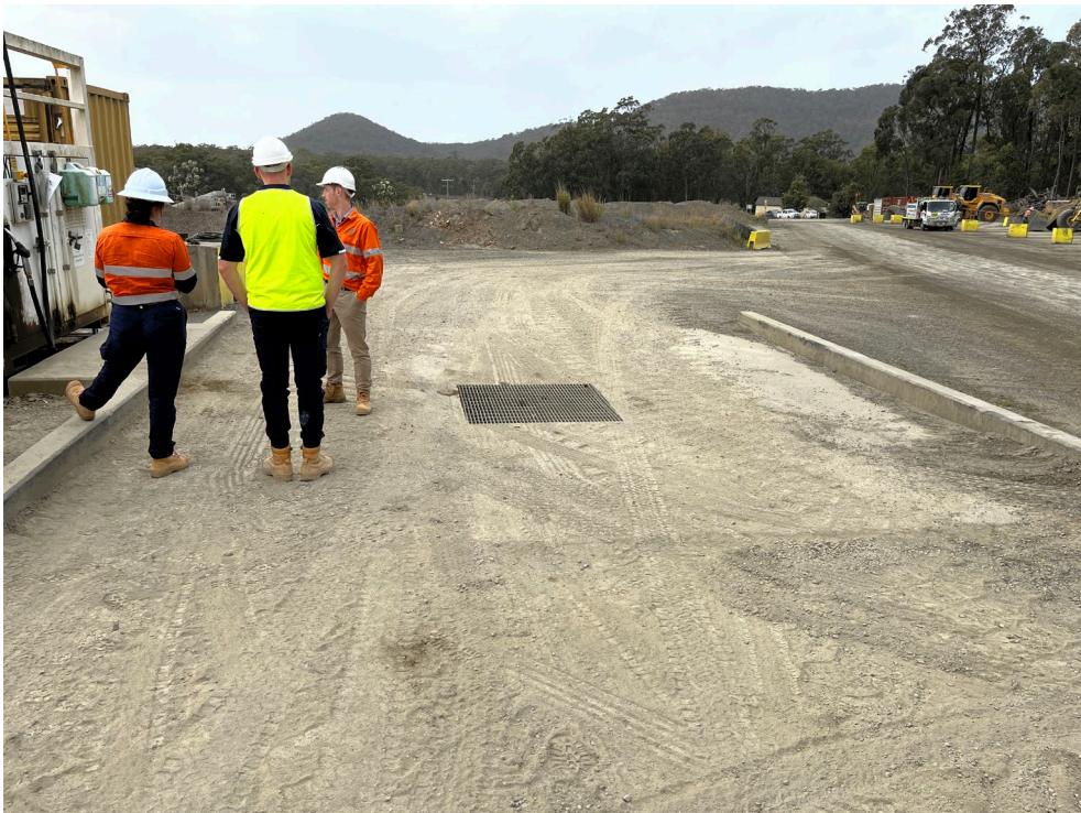
PHOTO 4 Refueling Hardstand and Sump
