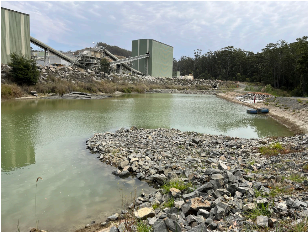
PHOTO 7 Surface Water / Sediment Dam
