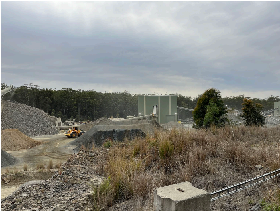
PHOTO 3 Sizing Plant (Cont.)
