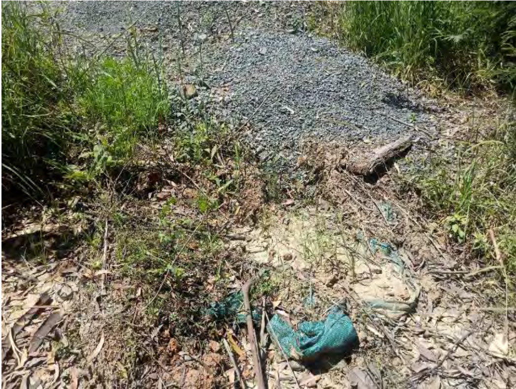
Photo 6: Sediment fencing down and overtopping within Lot 12.
