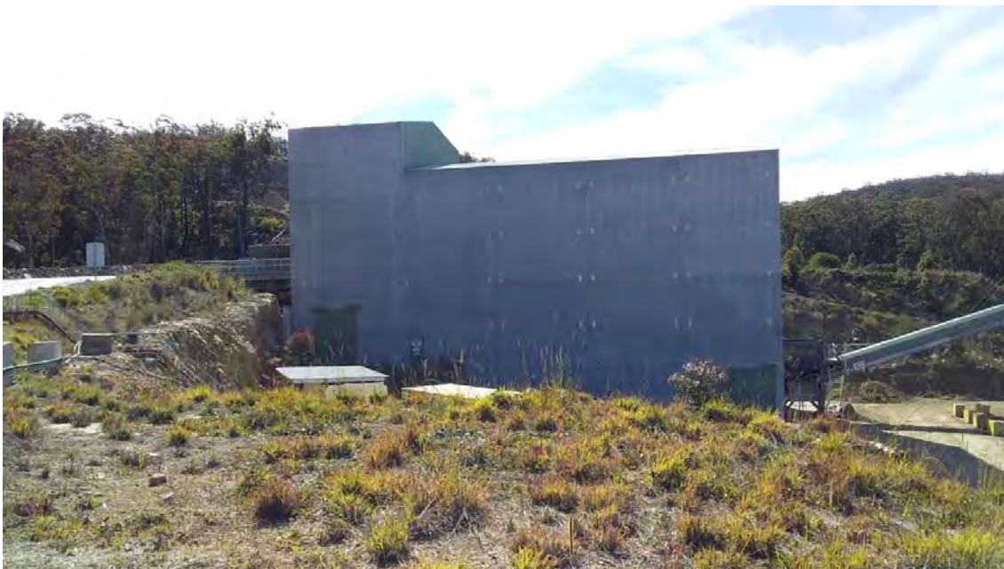
Plate 18 Enclosure of the site primary crusher to minimise noise and dust impacts
