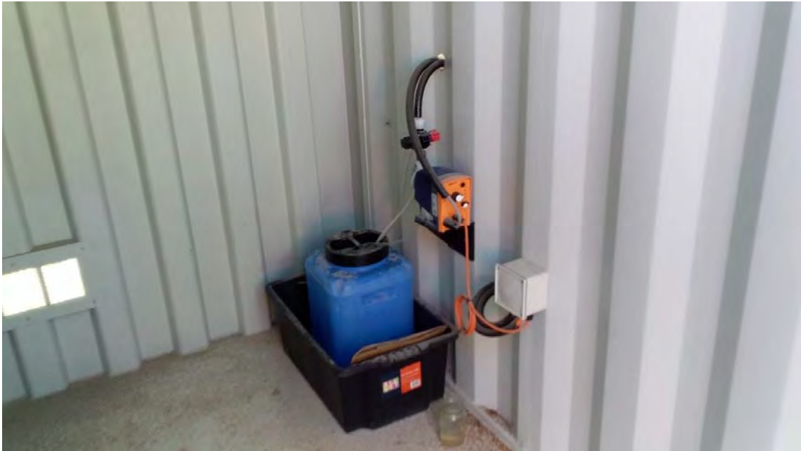
Plate 9 Dam 1 Flocculant Treatment System
