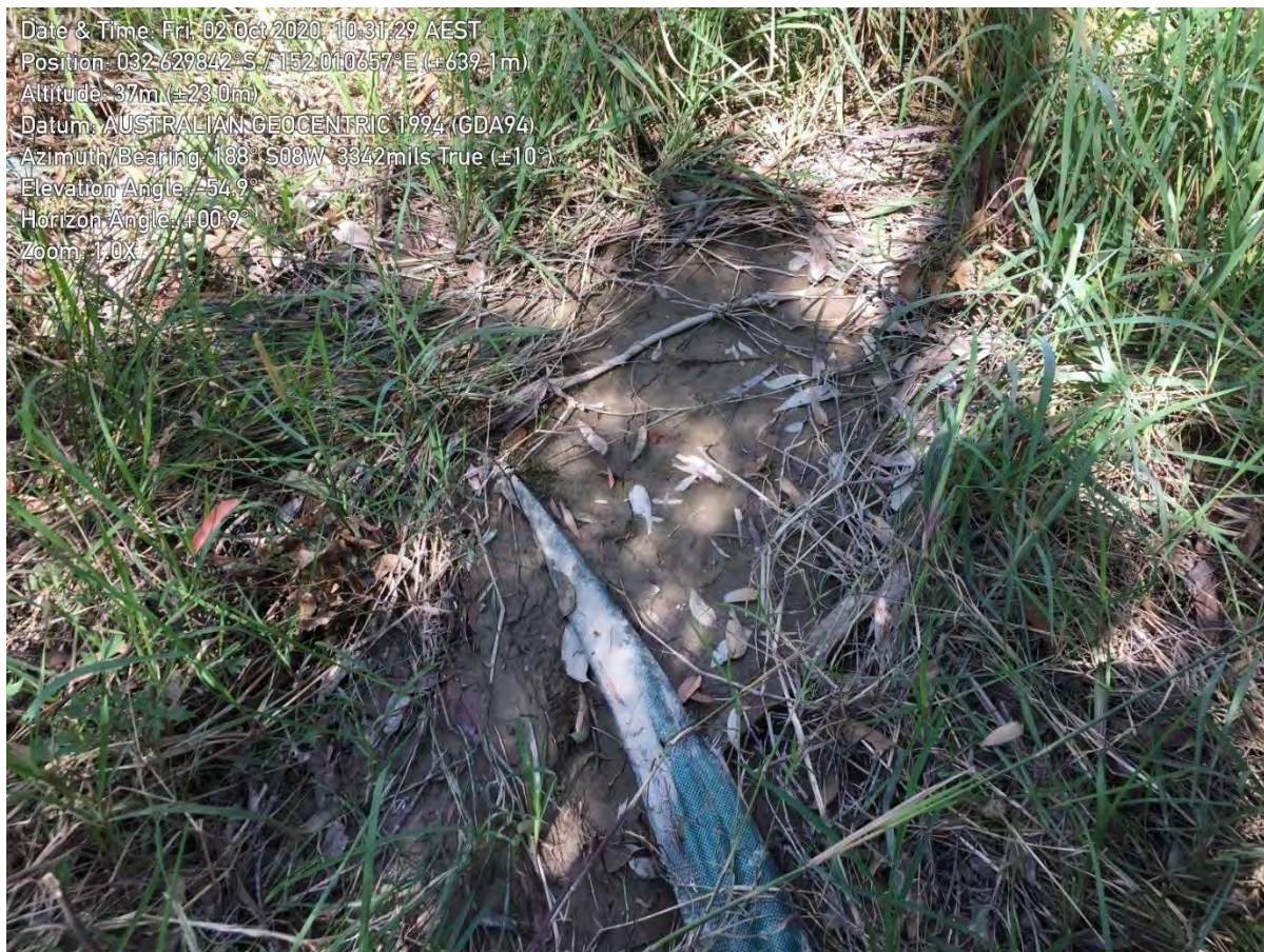
Photo 3 Sediment fencing down and overtopping within Lot 12
