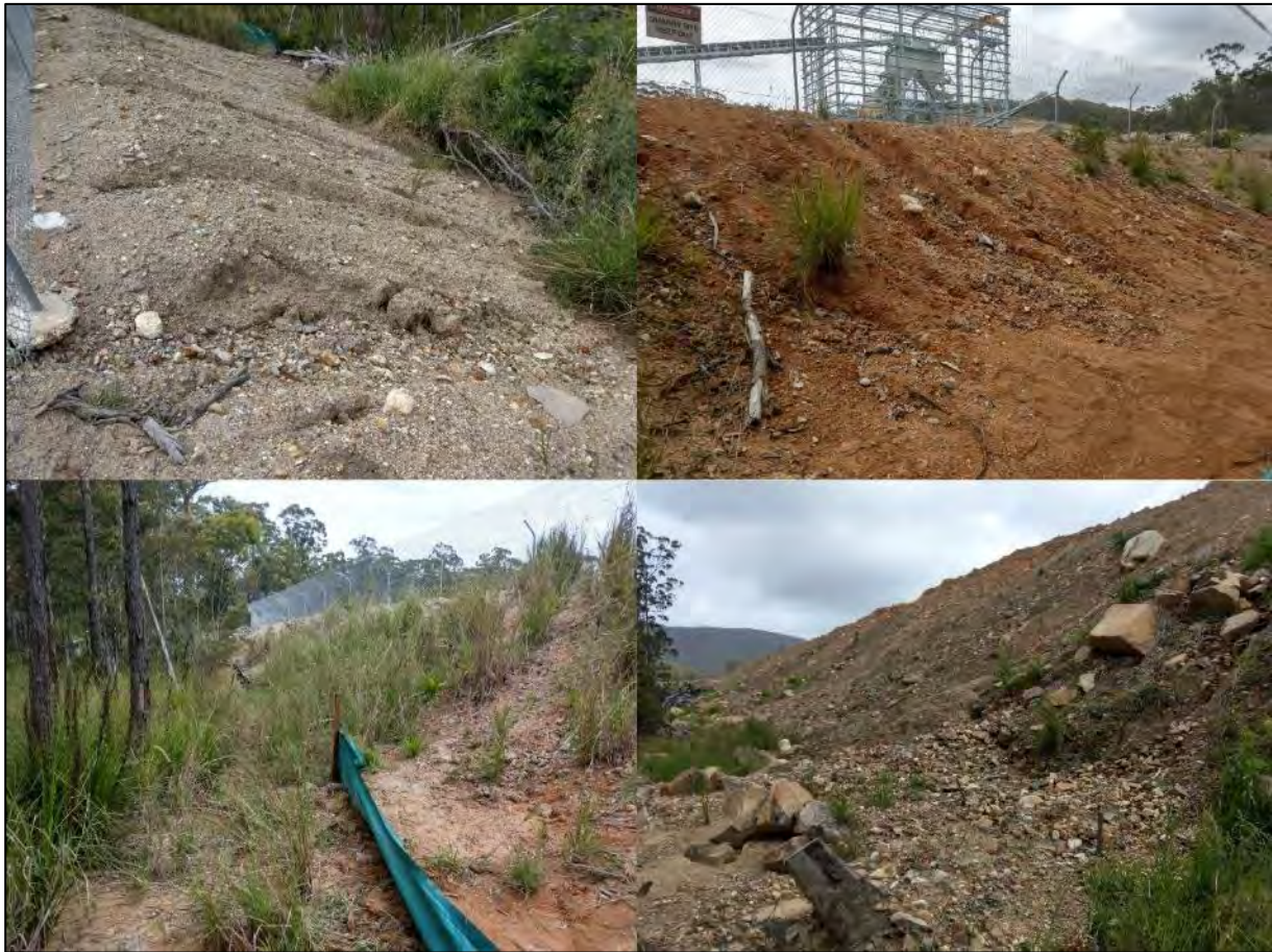
Plate 2: Erosion along the south-eastern bank of Dam 1 (top and bottom left) and the overburden stockpile (bottom right)
