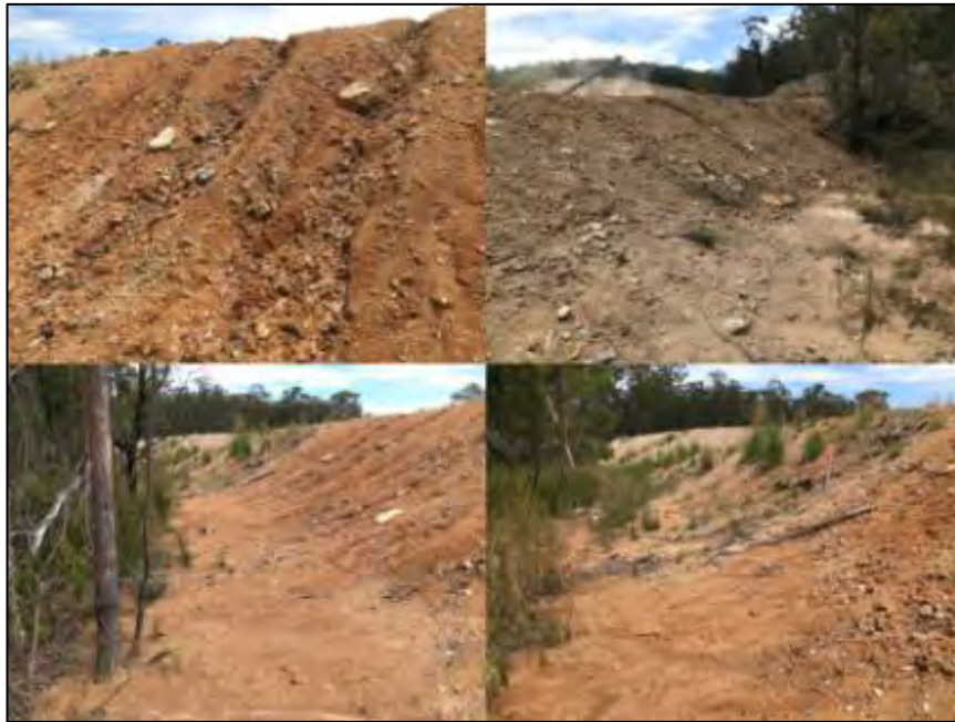
Plate 2: Erosion along the south-eastern bank of detention basin
