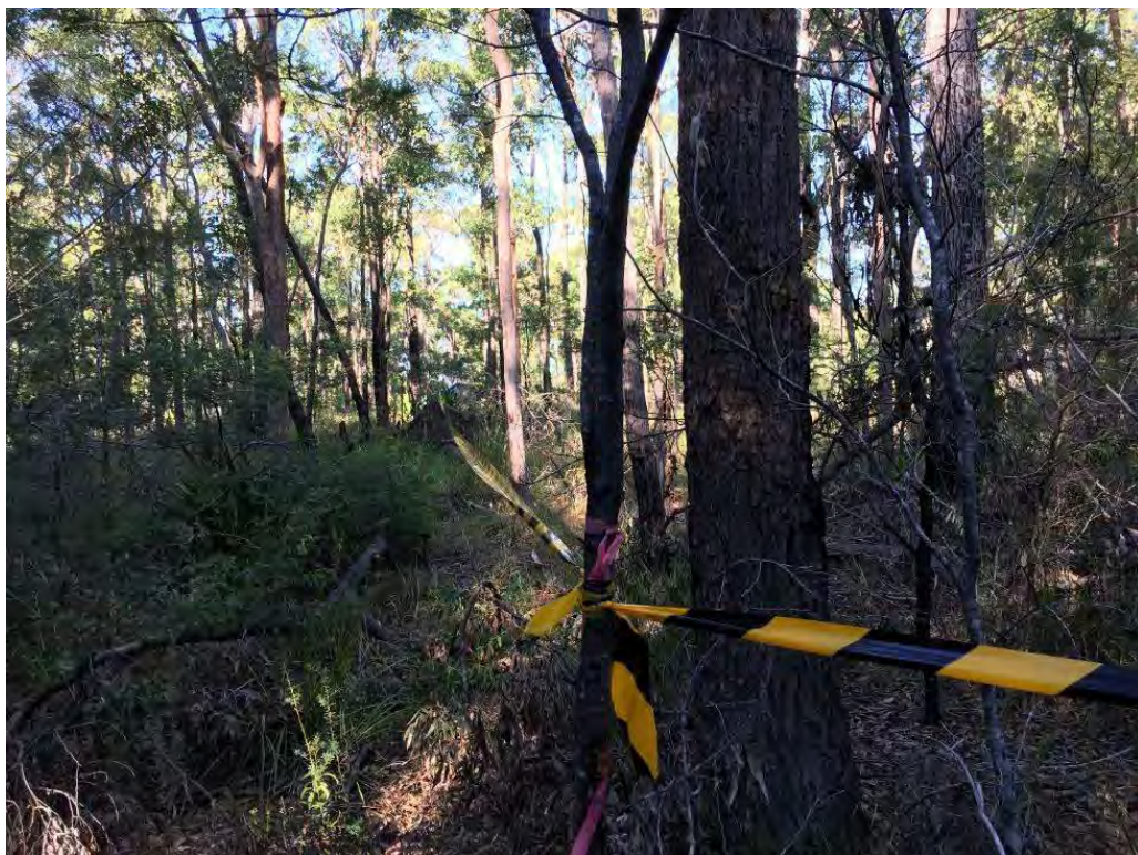
Photo 1 - Barrier tape and pink flagging tape is used to define the boundaries during the clearing process
