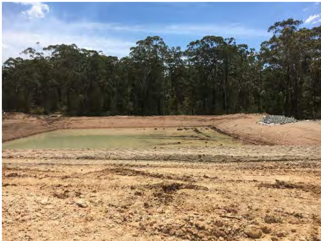
Photo 4 - Dam 3 - Spillway can be seen on the right
