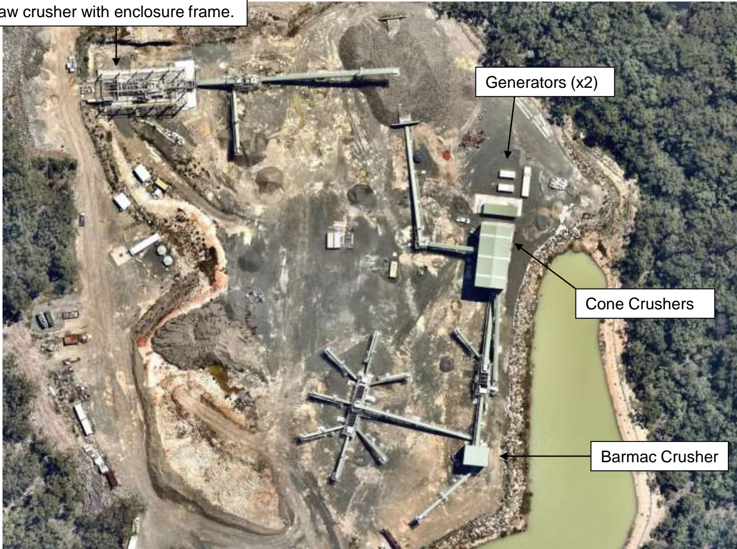
Crushing plant as of 14 February 2019
