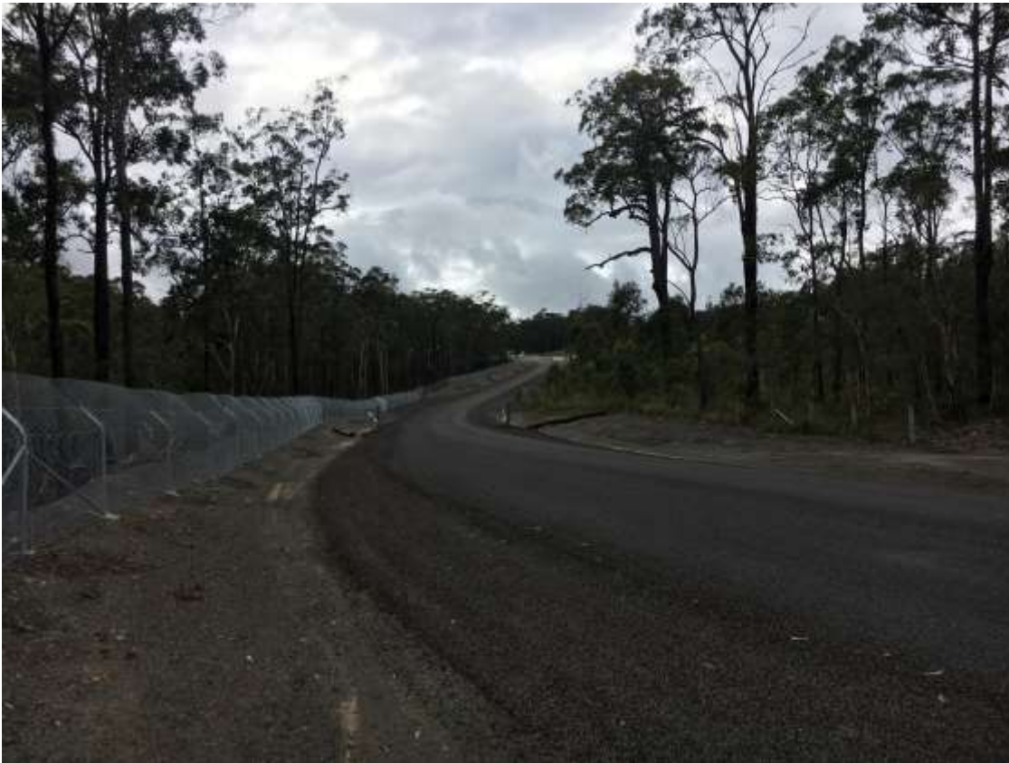
Internal access road looking towards the weighbridge from the entry. Chain-wire fauna fencing shown to the left. Photo taken 13 November 2017.
