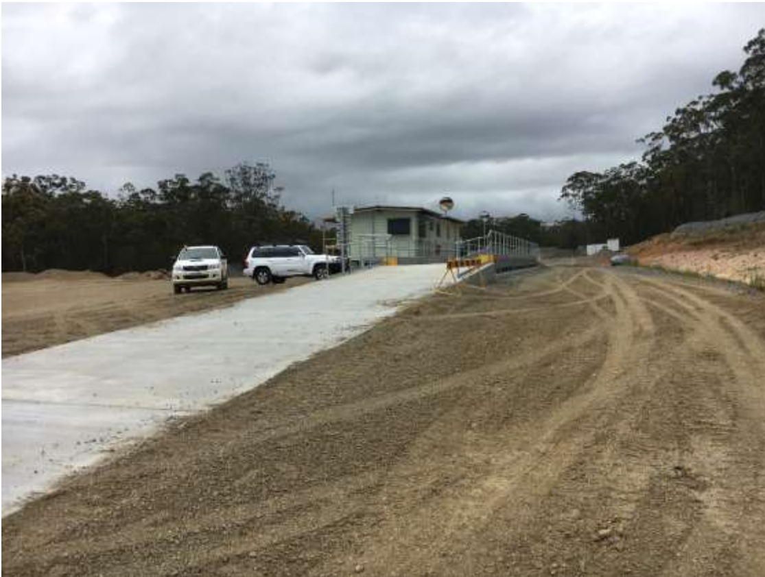
Weighbridge and office. Photo taken 13 November 2017.
