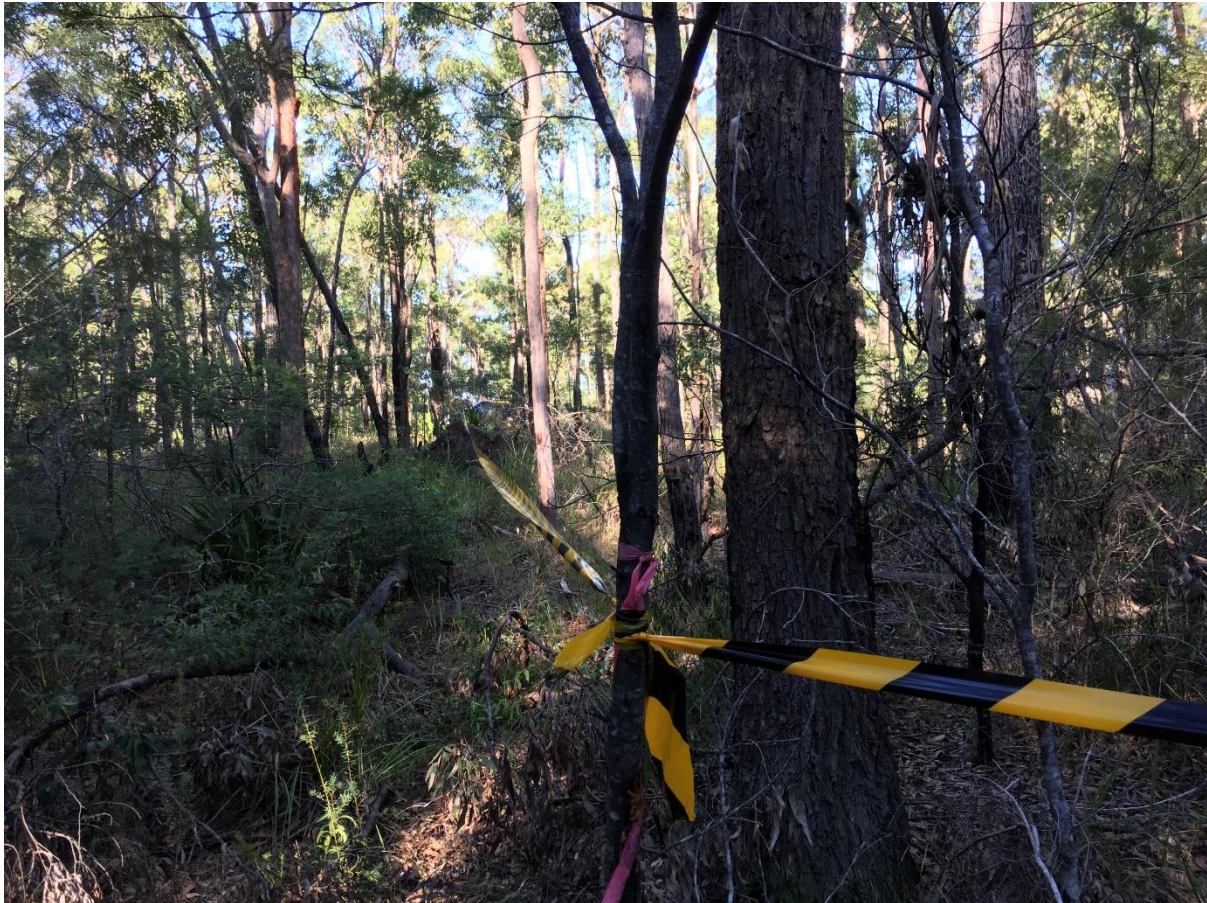
Barrier tape and pink flagging tape is used to define the boundaries during the clearing process.
